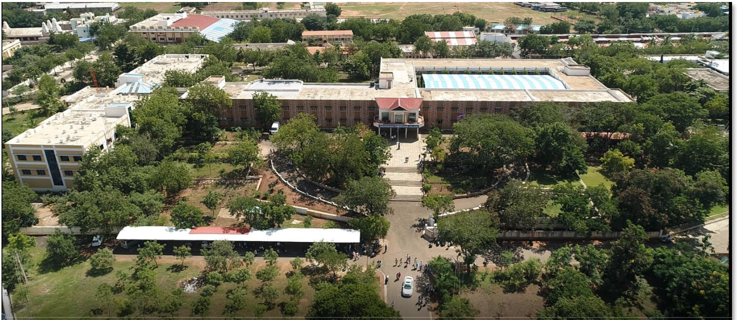
BEC- An aerial view
